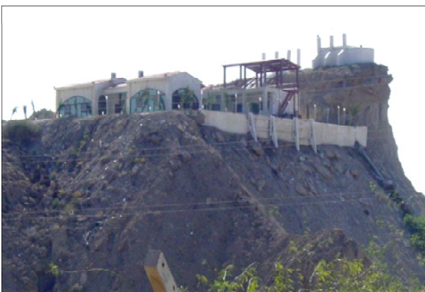
Figure 4. Fall in discordant slopes occurred by differential erosion of sensitive formation.
