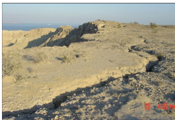
Figure 7. Wide crack tensions along the cliff edge of wave-built terraces formed in upper hard layer.
