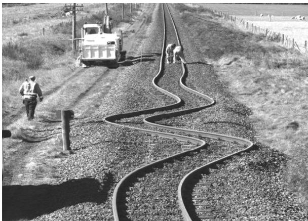
**Figure 5.** Photograph of a buckled track from [www.modernghana.com/news/305521/1/earthquake-twists-railway-tracks.html](http://www.modernghana.com/news/305521/1/earthquake-twists-railway-tracks.html).
