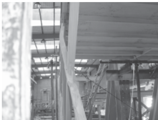
a) Buckling of the Compressive Bracing of the Second Specimen
