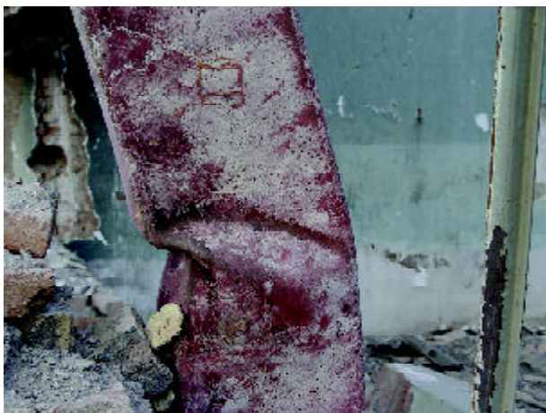
Figure 2. Local buckling of box column.
