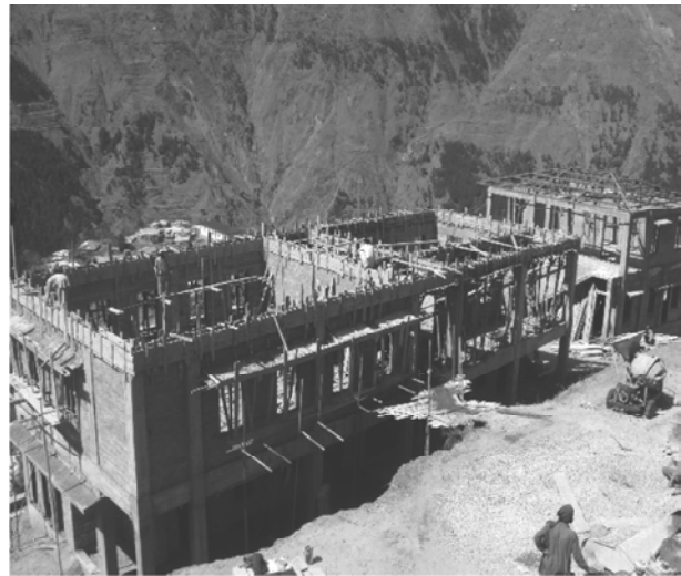
Figure 10. Construction of government boys schools, old Balakot peripheral development project .
