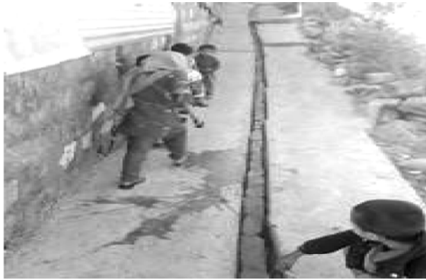
Figure 9. Improved streets and drainage, old Balakot town.
