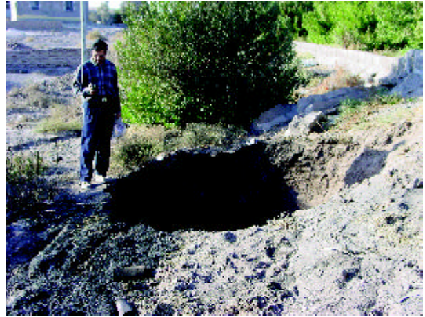
Figure 20. Sinkhole observed close to the main road of Bam to Zahedan near Baravat: same sinkholes induced under the road at the time of earthquake that affected the access of rescue and relief teams to the region.
