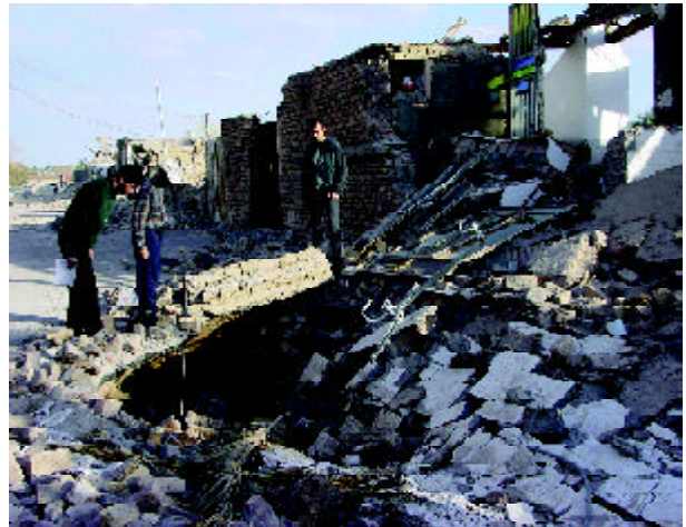
Figure 21. Damage to a building due to collapse of an old hidden Qanat (Baravat).
