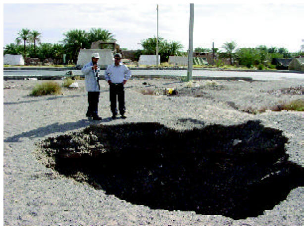
Figure 17. Large sinkhole observed at west of Baravat.
