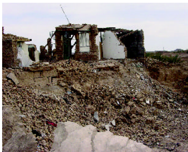
Figure 30. Damages to a building located at top of an excavation due to landslide, Esfikan village, Northeast of Bam.
