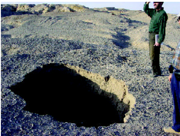
Figure 13. Sinkhole induced due to the collapse of a Qanat gallery; west of Baravat
