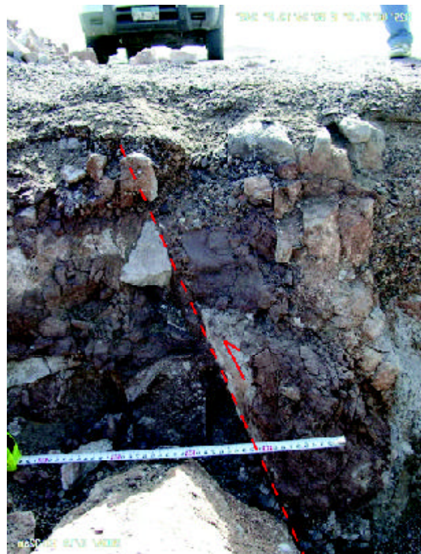
Figure 2. Erosion and weathering in Andesite and Basalt at the vicinity of Bam fault.
