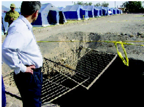
Figure 16. Large sinkhole; south of Bam.
