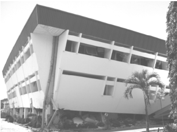
Soft Storey Mechanism [2]
