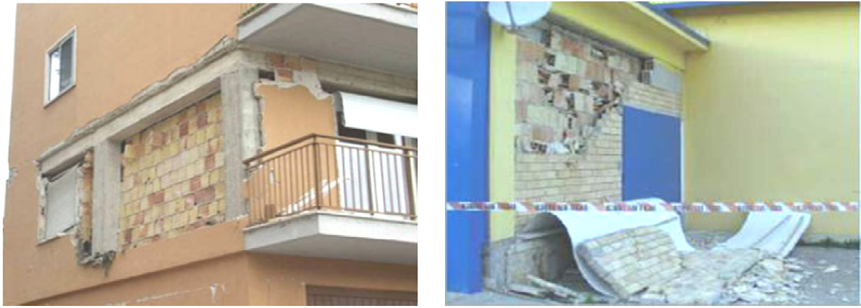
Figure 3. Detachment of the leaves in multi leaf walls [6].
