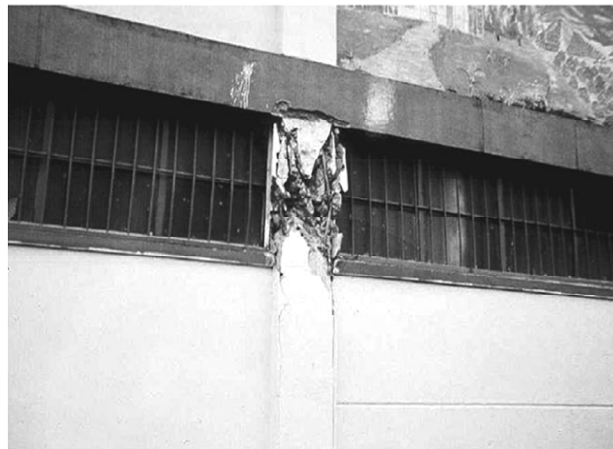
Short Column Mechanism [3]
