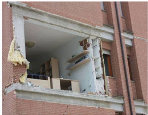
Figure 2. Damage in non-structural elements [6].
