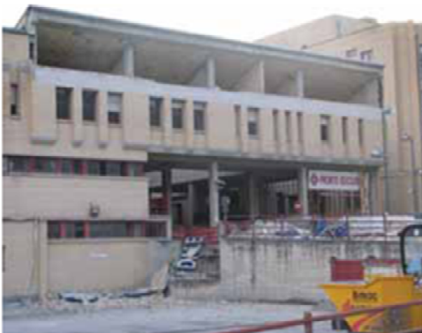
Figure 2. Damage in non-structural elements [6].
