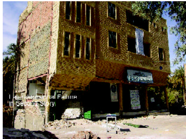
Figure 7. Eastern view of the insurance building.
