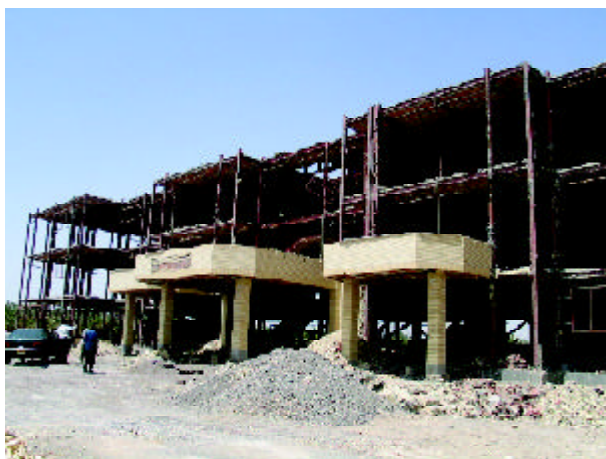
Figure 15. Southern view of nursery building.
