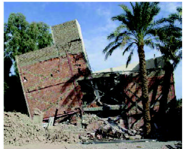
Figure 4. Southern view of Kimia building
