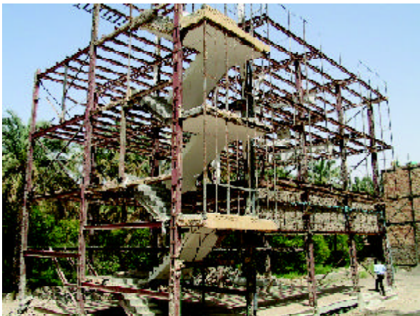
Figure 10. Demolition of the insurance building.
