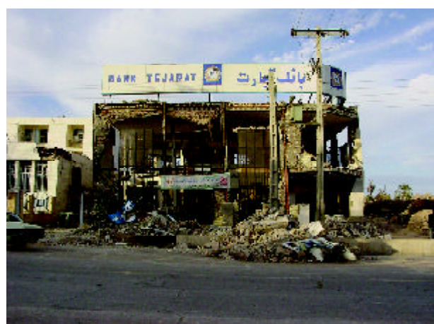
Figure 19. Southern view of bank Tejarat.
