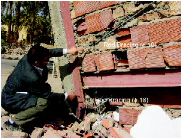
Figure 5. Rod bracings in stories.
