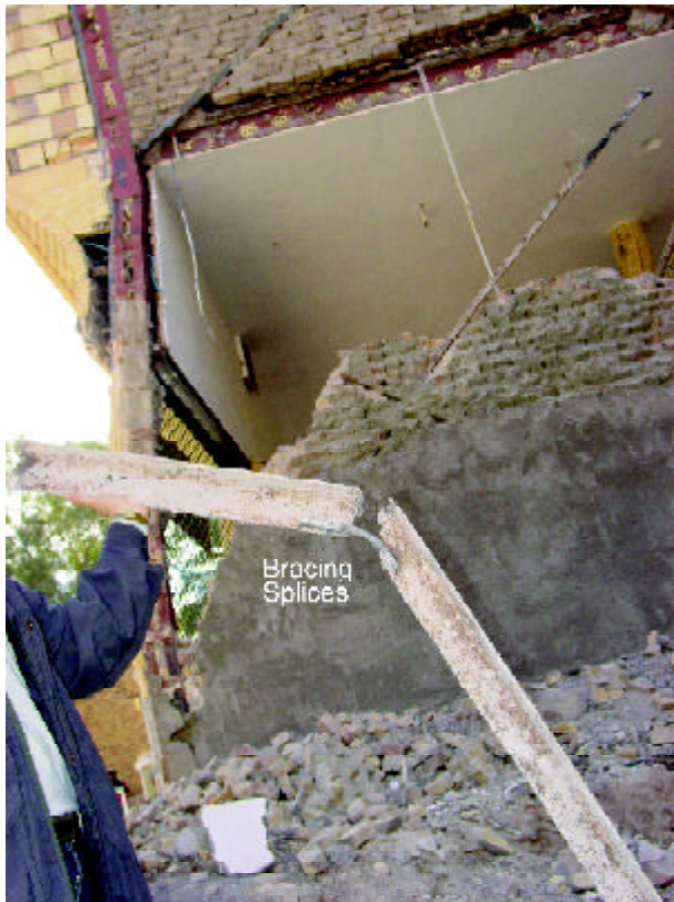
Figure 9. Brace spliced with a rod.
