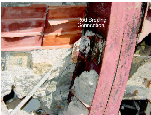
Figure 6. Rod bracing connections.
