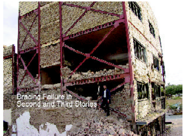
Figure 11. North view of the residential building.
