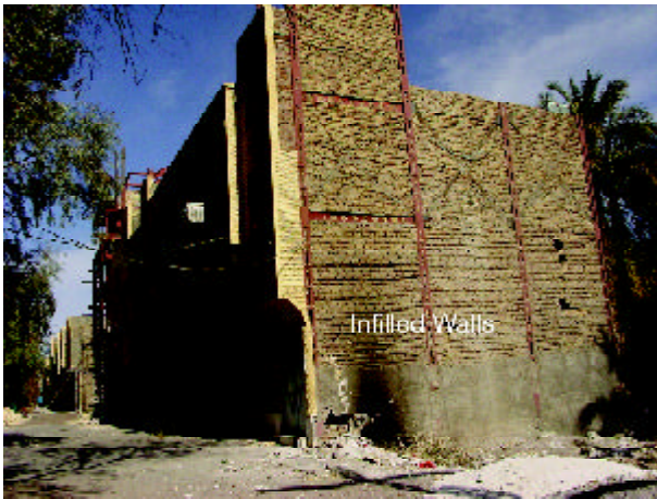
Figure 25. Masonry infill building.
