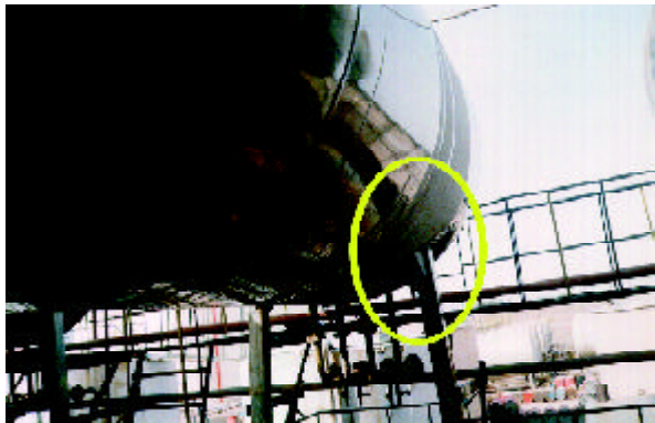
Figure 22. Punching of tank shell [1].
