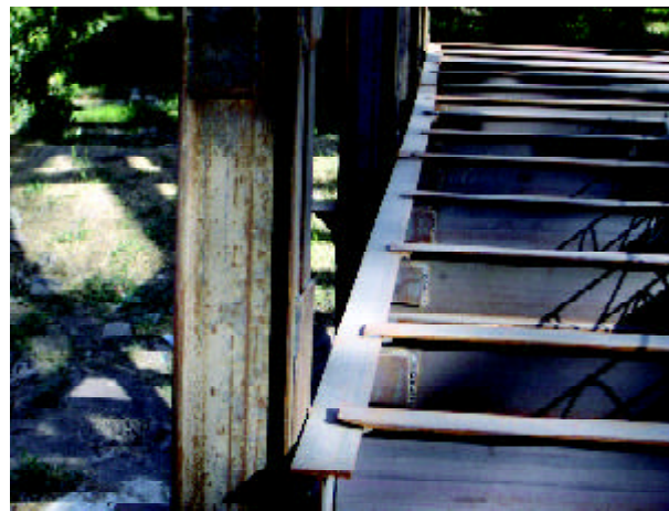
Figure 1. Commonly used jack arch slab (left: wall supporting, right: girder supporting).
