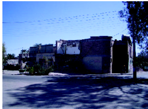
Photo 1. North view of Governor's building.
