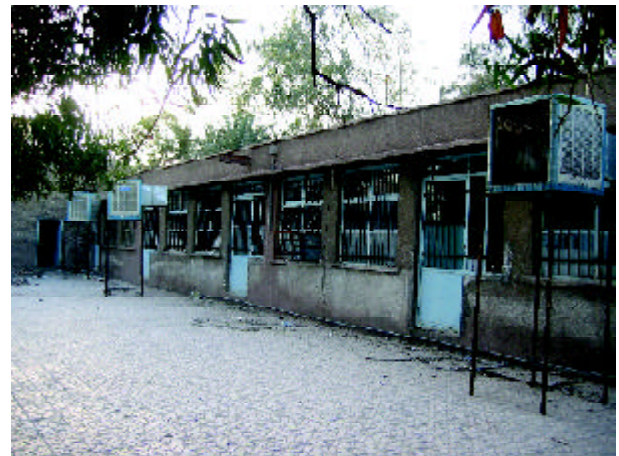
Photo 5. Single-story school building (slight damage).
