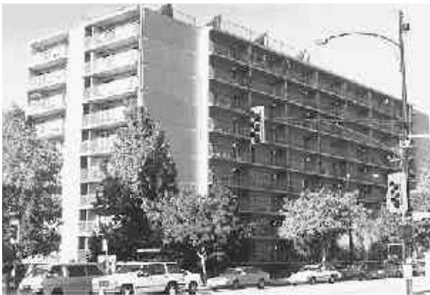
Figure 10. General view of 10-story residential building in Burbank [24].
