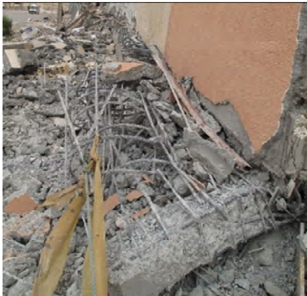
Figure 37. The inadequate anchorage of longitude reinforcements in Eslamabad-e Gharb, Mehr buildings.
