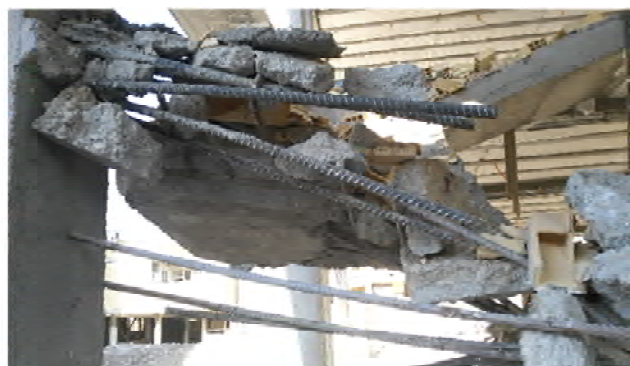
Figure 16. Pulled out bars because of ignoring the standard bending of bars at the conjunction of the staircases and columns.
