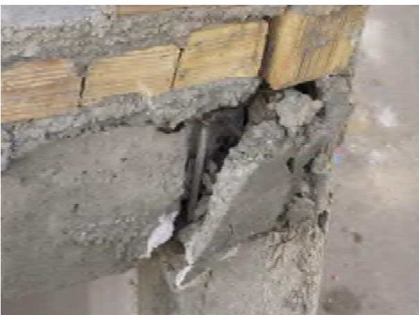
Figure 29. Imperfection in using 90 degree hooks at the end of the longitude bars.
