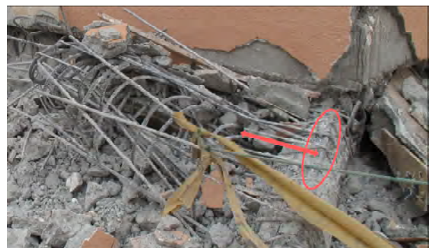
Figure 37. The inadequate anchorage of longitude reinforcements in Eslamabad-e Gharb, Mehr buildings.
