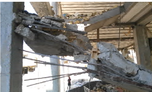
Figure 16. Pulled out bars because of ignoring the standard bending of bars at the conjunction of the staircases and columns.
