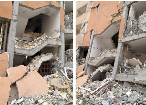
Figure 15. Staircases separated the structures at the level of first floor.
