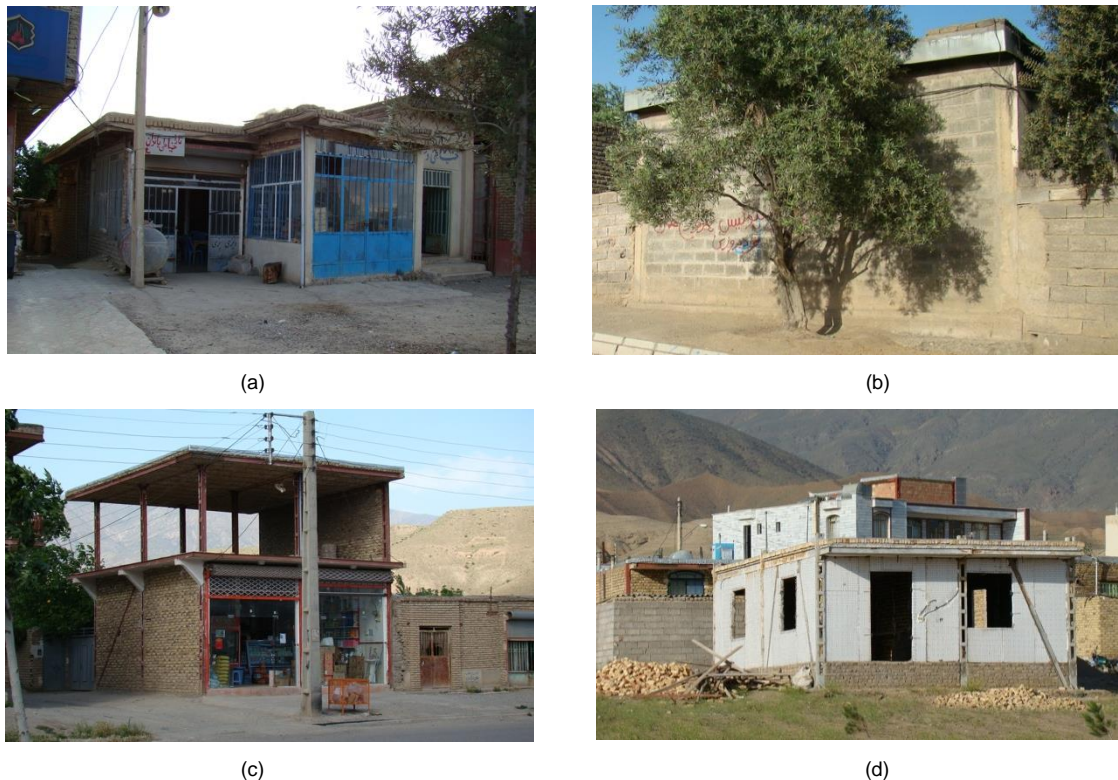
Figure 9. Sample of observed buildings in cities in different construction period. a) A vulnerable steel structure without any proper lateral resistant system; Constructed in reconstruction period, considered as vulnerable structure. b) Confined masonry structure with proper vertical and horizontal ties; Constructed in reconstruction period, considered as a safe structure. c) A steel structure with lack of bracing in second floor and vertical irregularity; constructed in developing period and considered as vulnerable. d) A well-constructed steel structure built in developing stage, considered as safe.
