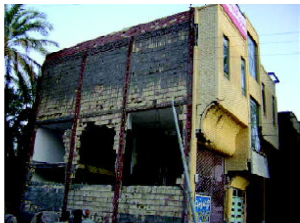
Figure 12. Simple steel frame without bracing.
