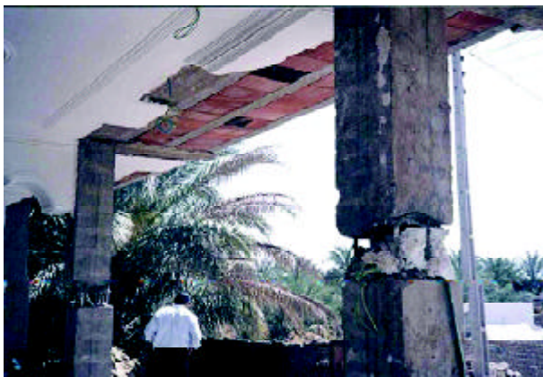
Figure 15. Removing concrete to install stair case.
