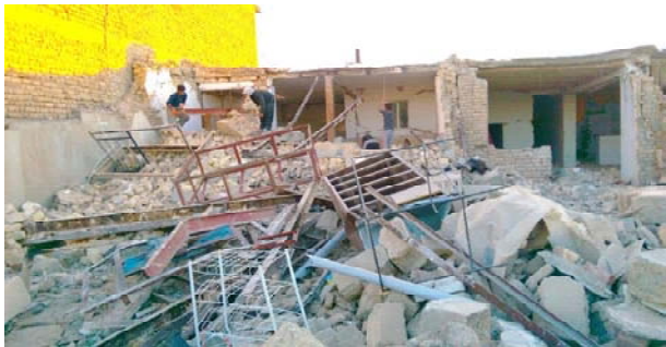
Figure 2. Some of the collapsed buildings of Ghara-Belagh-Azam.
